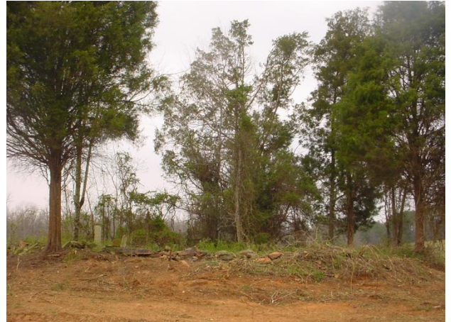
This is the after shot, taken about 3:00 pm. We are a little over half way finished, a great more deal of work to do.
