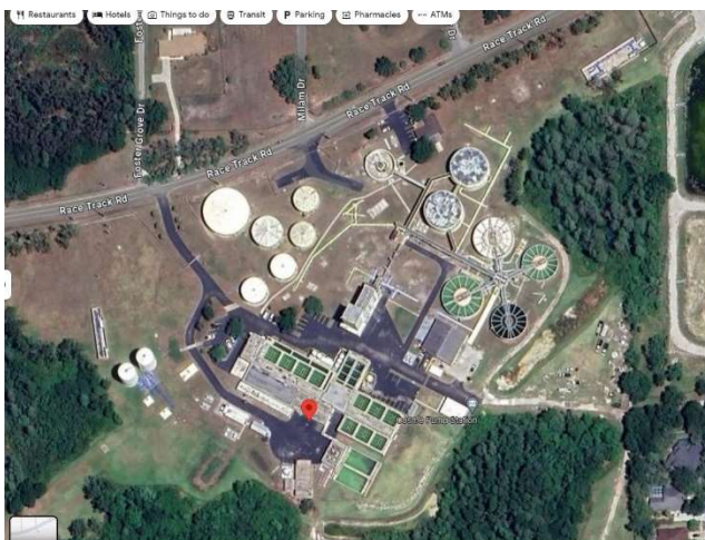
Cosme Saint Petersburg water treatment plant located in Odessa, FL. 16015 Race Track road
