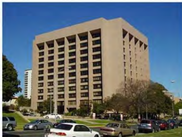
Stephen F. Austin State Office Building
