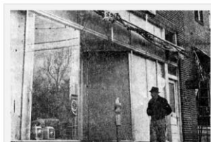
A man walks by the boarded-up window in the store front of Western Auto on Locust Avenue after the dynamite explosion.
